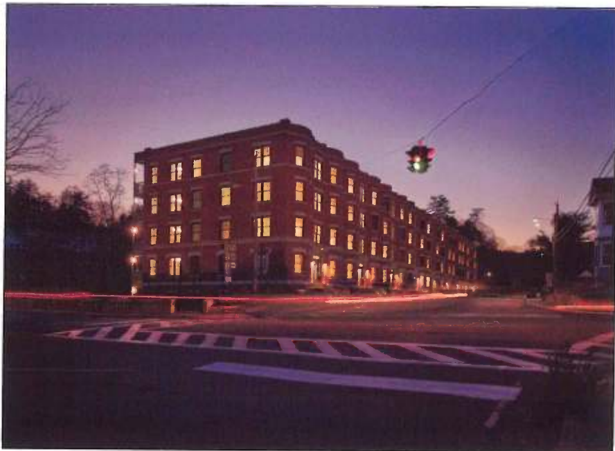
Union Square Apartments, Windsor Gut rehabilitation to create 58 family apartments
