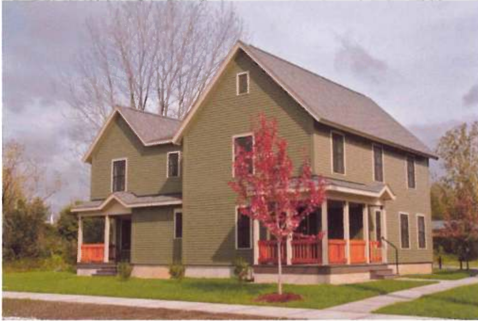
Hickory Street, Rutland Redevelopment of former Forest Park Public Housing 56 apartments and community space in two phases
